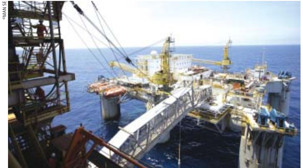
MAN Diesel & Turbo SE has concluded a long-term service agreement with the Brazilian energy group Petroleo Brasileiro (Petrobras) for the maintenance, repair and operational support of 20 MAN THM gas turbine trains on four offshore platforms in the crude oil and natural gas exploration area off the north-east coast of Rio de Janeiro.
