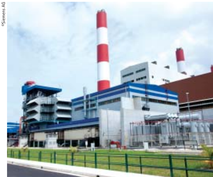
The PowerSeraya's 800-megawatt Combined Cycle Power CoGeneration Plant in Singapore built by an open consortium with Siemens AG as the consortium leader
