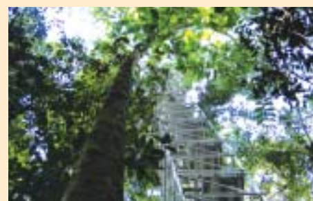
Two towers are already at the ATTO site. These 80 meter high towers have already been regularly collecting data on weather conditions, ozone, CO 2 volatile organic compounds and nitrogenous trace gases and aerosols since 2011.
