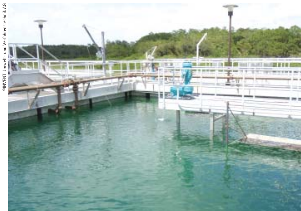
Energy-efficient INVENT hyperboloid mixers at the WWTP Bowery Bay in New York, USA
